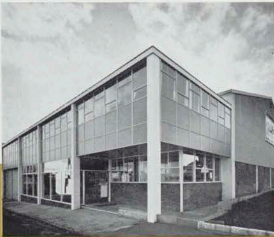
E. W. Pidgeon's warehouse and offices, Newmarket, Auckland. Architect: Kenneth Albert; Contract Manager: Bill Anderson; Foremen: Alex Noble and Norm Hansen.
