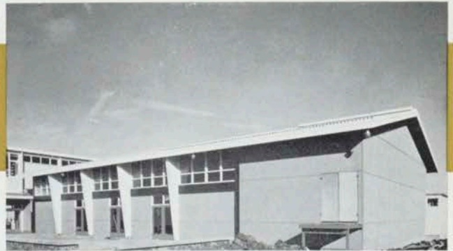
Penrose High School Assembly Hall. Architects: Ministry of Works; Contract Manager: Bill Anderson; Foreman: Trevor Horsnell.
