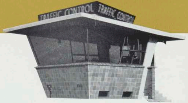
Auckland Harbour Bridge Authorities traffic control tower. Designed to house speed detection and closed-circuit television equipment. Architect: Llew S. Piper; Contract Manager: Bill Anderson; Foreman: Arthur Newton.
