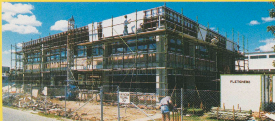
Office extensions for Glass Containers Ltd, Penrith, N.S.W.
