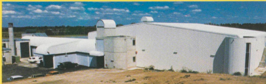
The recently completed extensions to the N.S.W. State Archives, at Kingswood.
