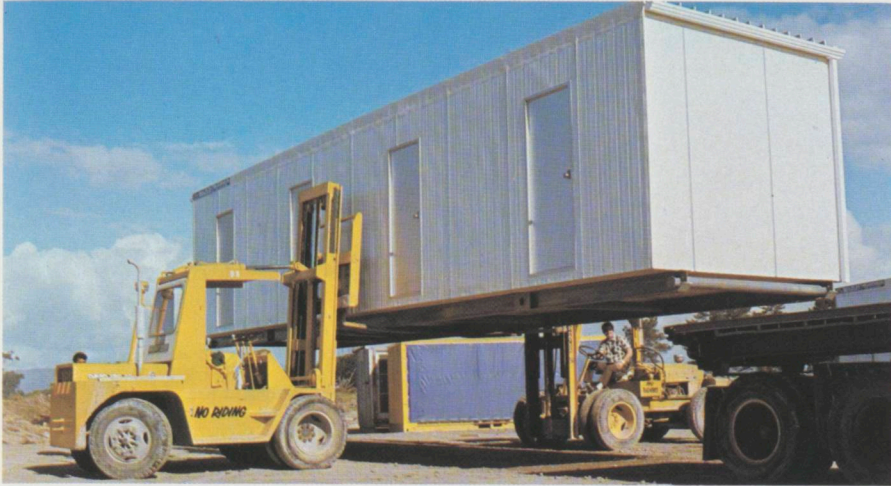
Unloading a four-man accommodation unit from its transporter. For shipment overseas, each unit is packed flat to make a package only 750 mm high.
