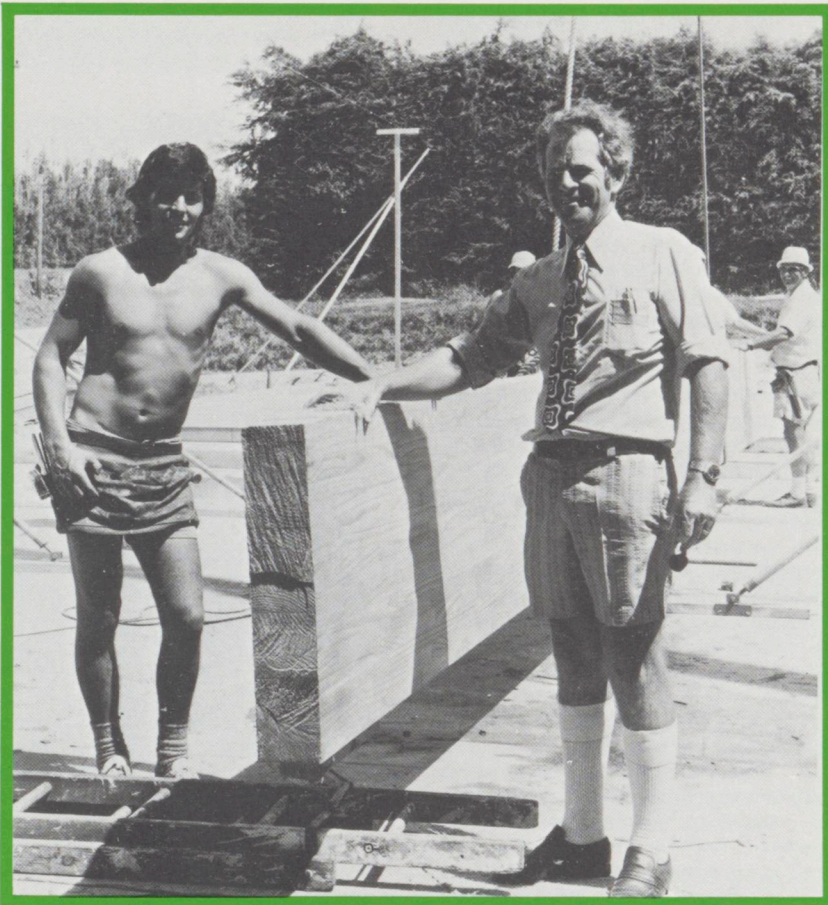
Builder Mr Paul Baigent (left) and Mr D. W. Ede of Fletcher Timber, Rotorua, with one of the massive laminated beams used in the packing shed.
