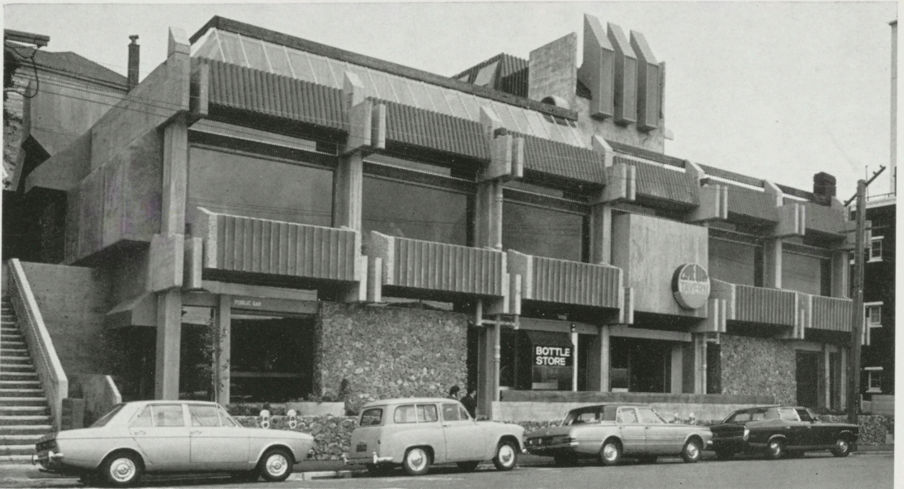
Clyde Quay Tavern, Wellington, built by Fletcher Construction, on a difficult site, is now open for business. An unusually interesting exterior is complemented by an interior which is colourfully attractive. Architects were the Pierce Group. Fletcher Construction Contracts Manager was J. S. Craig and Foreman R. Carr.
