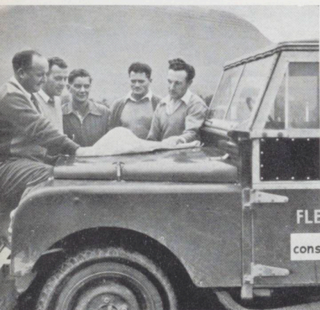
Jack Bourke (left) with housing foremen on the townsite.
