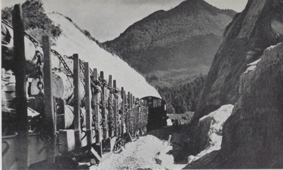
The first rail load of logs coming down the new line from the forest.
