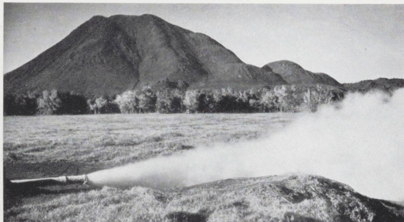
One of the smaller geothermal steam bores alongside the site at Kawerau.
