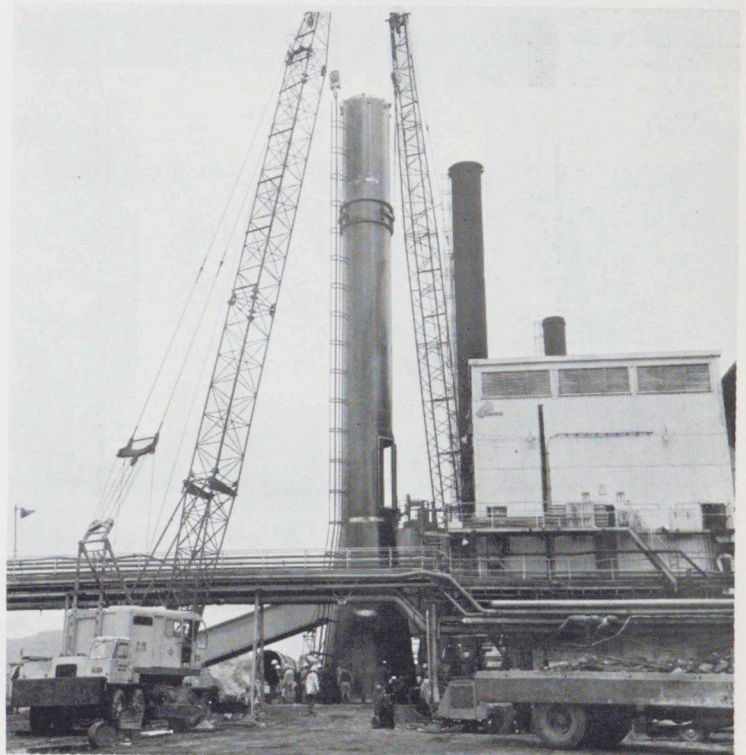
Above: The base section of the stack on its way up with the 20-ton truck crane drifting the base in over the foundation. Below: The base section in position and being bolted down. Below left: The same operation with the model.
