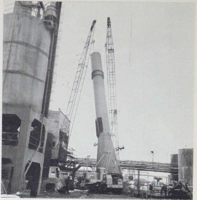
Above: The base section of the stack on its way up with the 20-ton truck crane drifting the base in over the foundation. Below: The base section in position and being bolted down. Below left: The same operation with the model.
