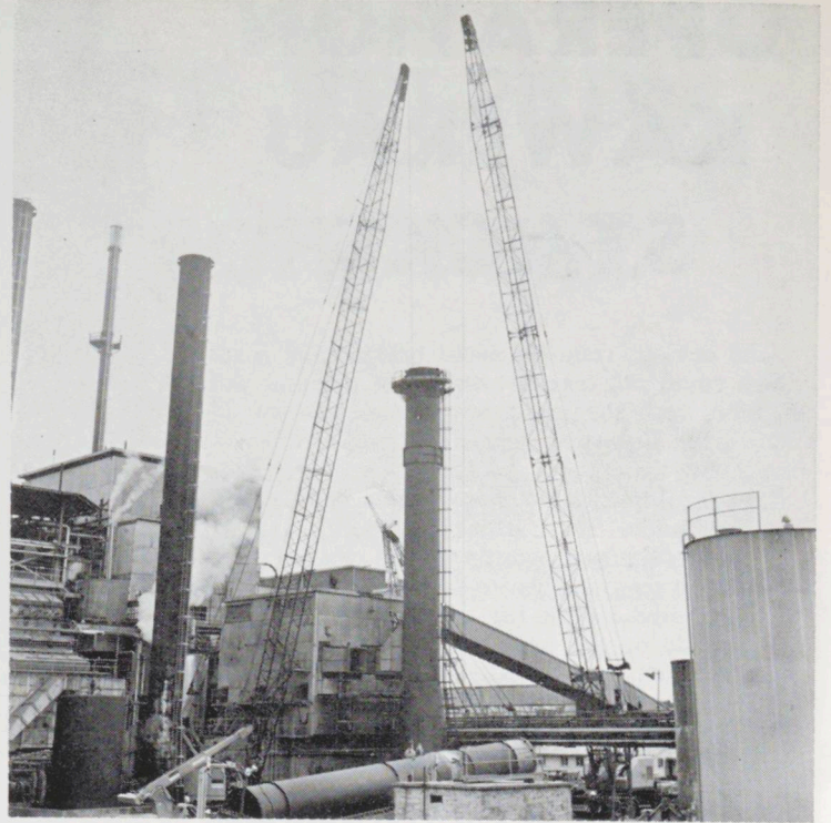
Above: Cranes in position with 170ft. and 180ft. booms ready for raising the top section; and model of the same operation. Below: Top section of the stack being assisted into position by the Austin Western crane.
