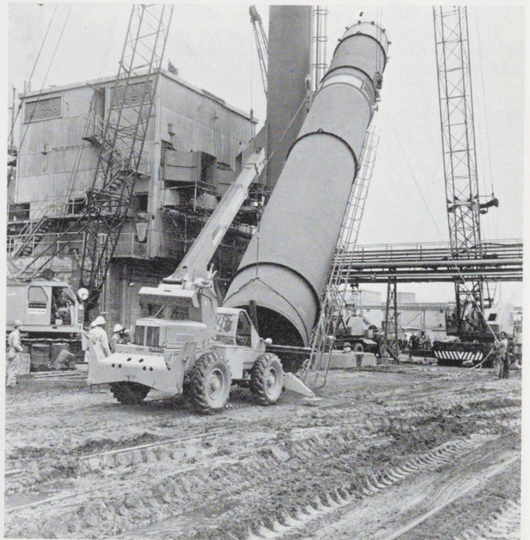
Above: Cranes in position with 170ft. and 180ft. booms ready for raising the top section; and model of the same operation. Below: Top section of the stack being assisted into position by the Austin Western crane.
