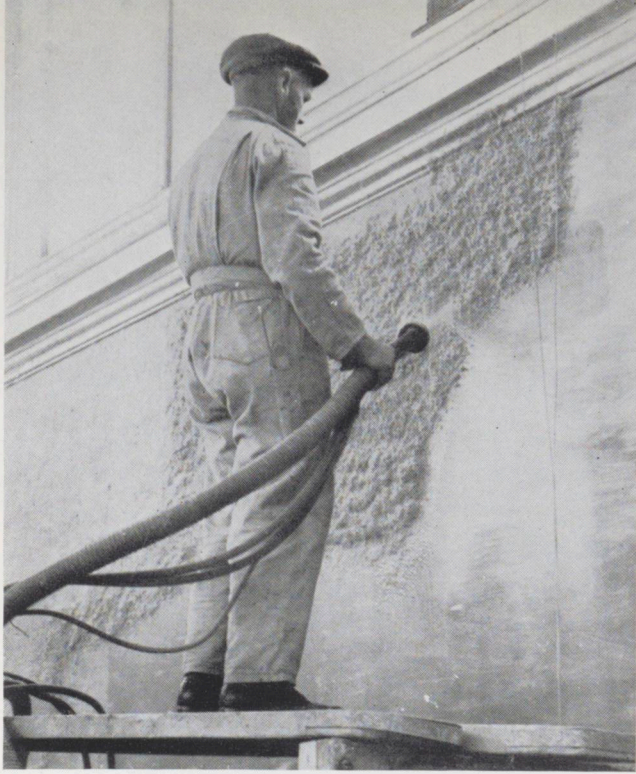
Sprayed "Limpet" asbestos being applied at Law Courts, Oamaru.
