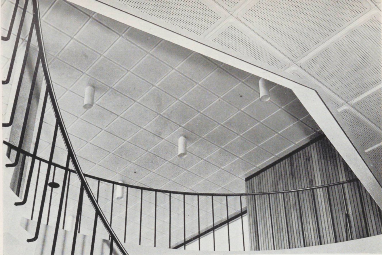
Otago University Library — some of the 23,000 acoustic ceiling tiles (above), and (below) a section of the 3,500 yards of Par-K flooring.
