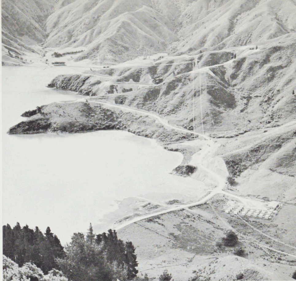
Hakana Bay near Port Underwood, with the camp built for the construction workers.
