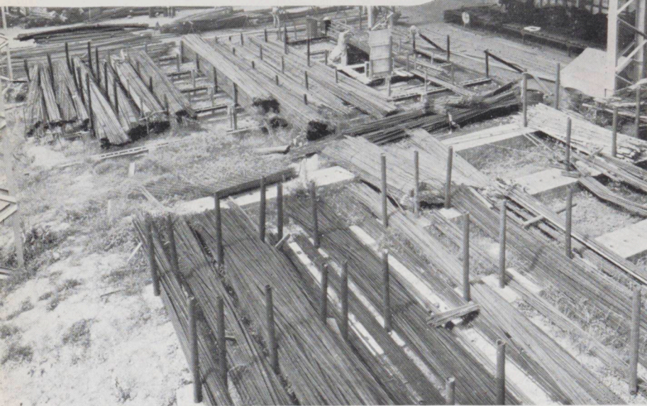
The structural steel workshops and reinforcing steel yard at Nelson Street.
