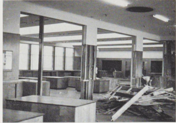
Down comes the main partition which divided the office into two large rooms.
