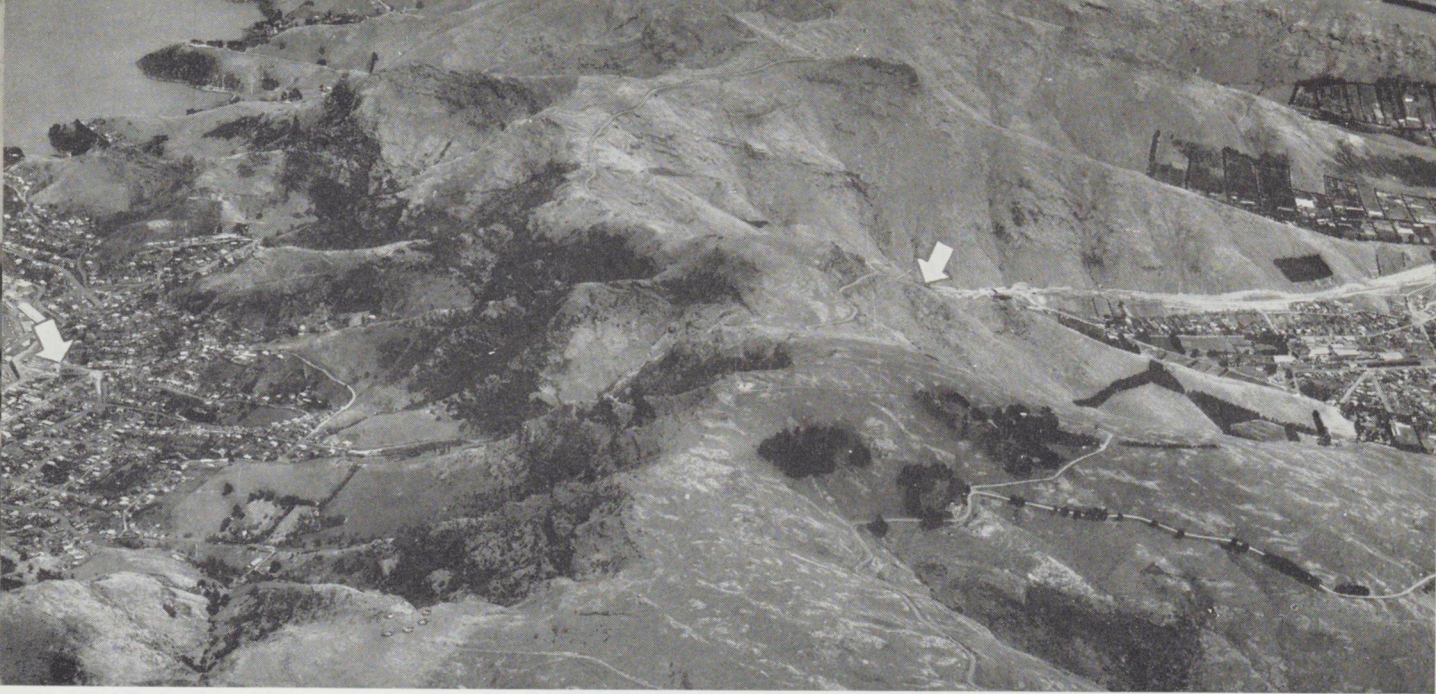
An aerial view of the Port Hills with arrows indicating the entrances to the tunnel.
