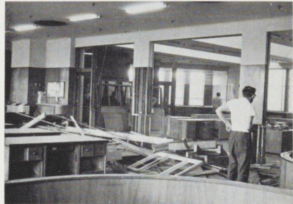
Alex Marks surveys the wreckage during the gutting of the offices.
