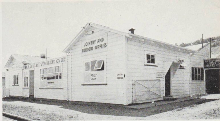
Head Office, Taitua Street, Taumarunui.
