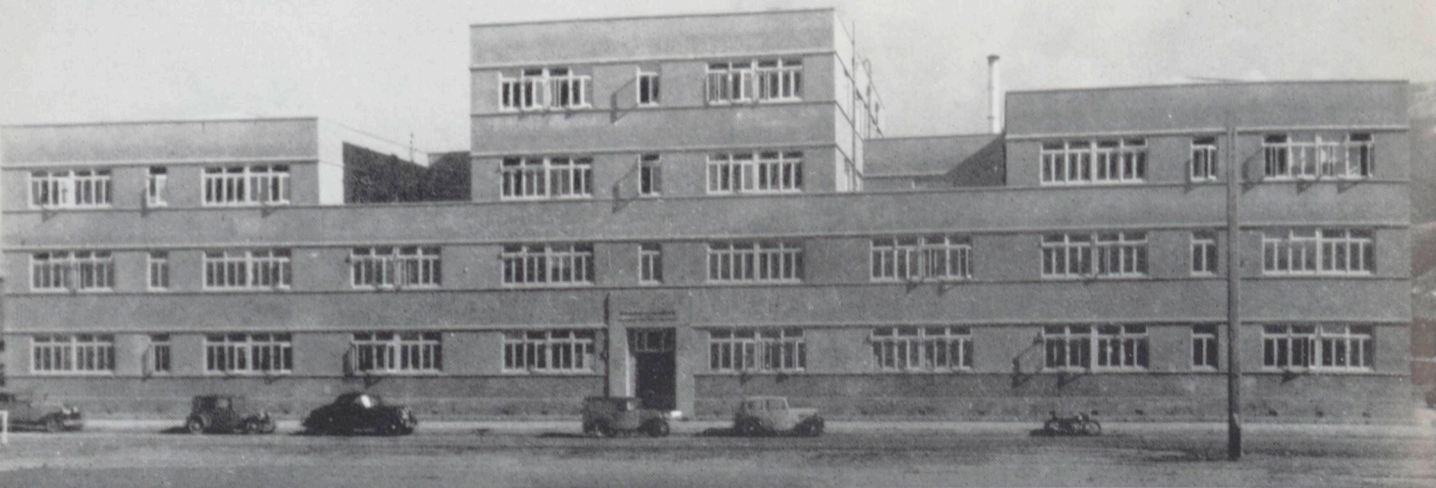
The completed building for the Social Security Department on Aotea Quay, Wellington, erected and fully finished inside six weeks.
