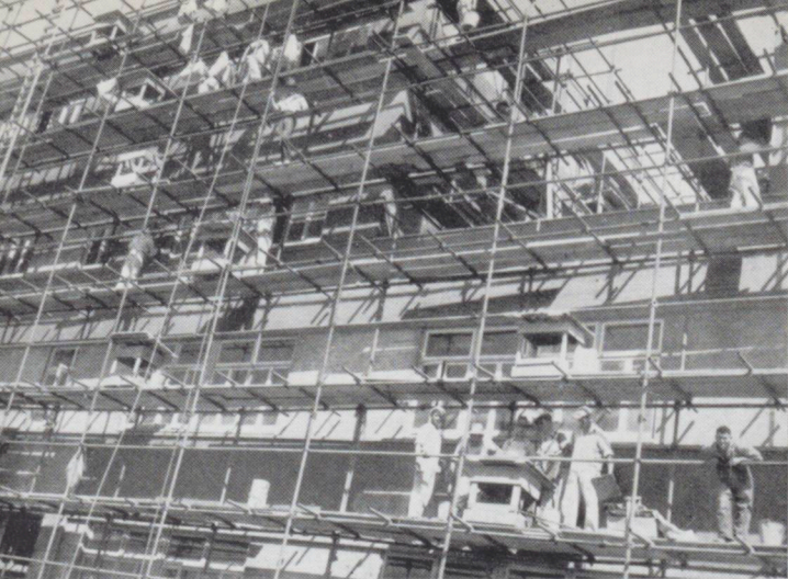
The big team of plasterers at work on the rear elevation.
