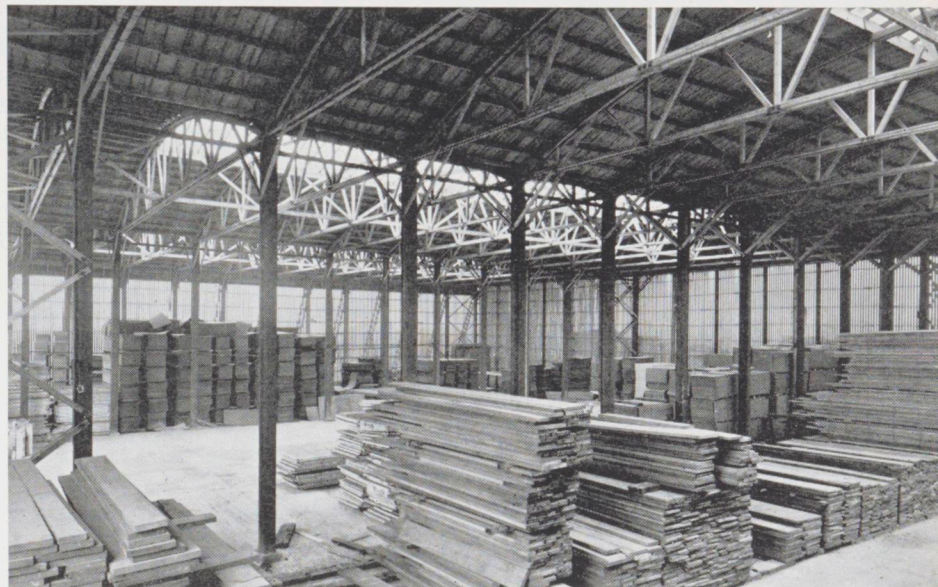
Top and bottom chords of glue-laminated timber are a feature of the bowstring trusses in this modern timber-drying shed built in England. The spans are 66 feet.
